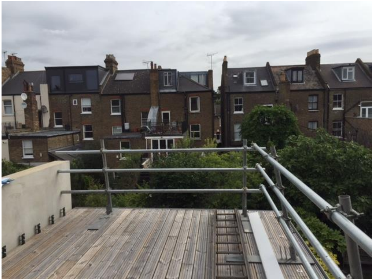
Image 4. – View of existing flat roof
