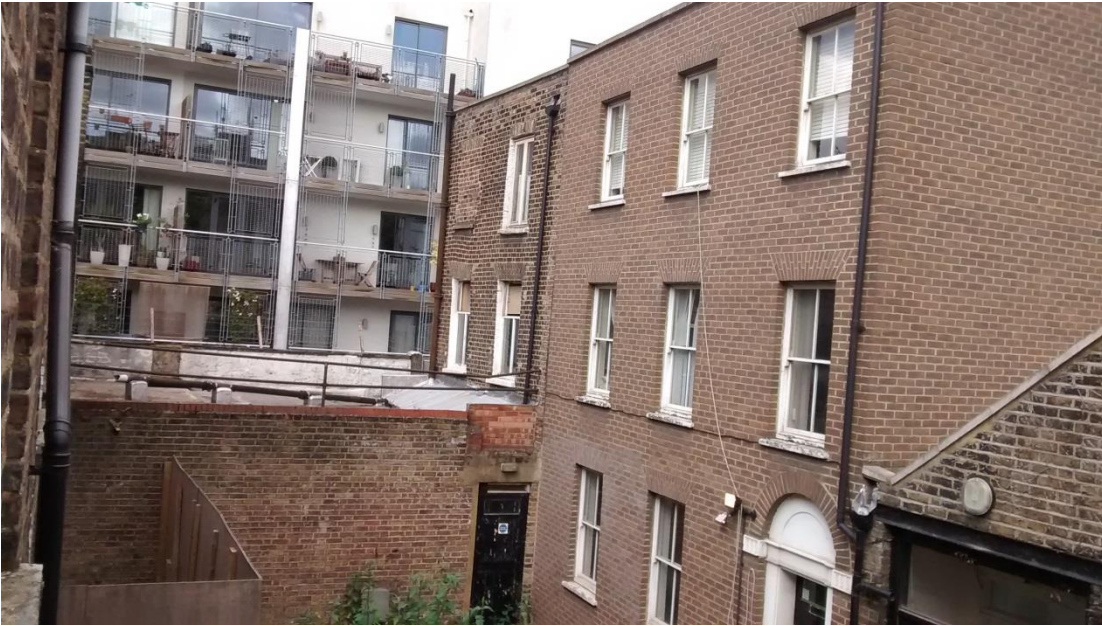
Image 5: View of the interior of the site from the first floor of 114a Pentonville Road
