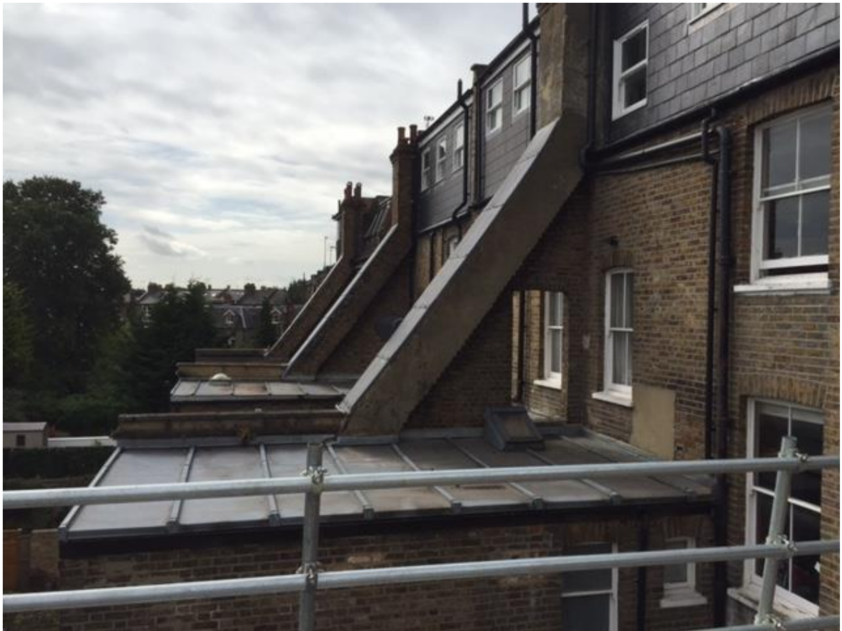
Image 5 – View from flat roof
